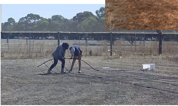
Setting up an irrigation system
